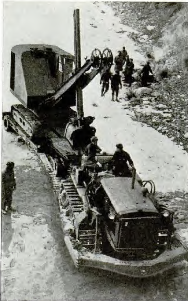
Somewhere in the winterbound wilderness a big shovel gets a lift from a tractor. The pioneer road is to be finished in a year
